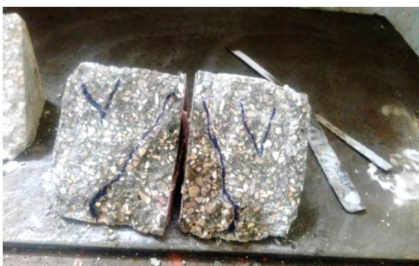
Fig. 10. Water penetration depth
